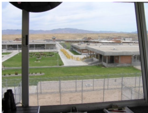
A view from one of the rooms at Tower 1 of Idaho State Correctional Institution
